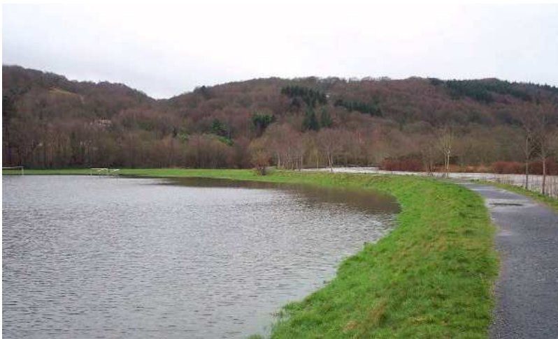
Figure 3.121: Flooding of the Marian Mawr playing fields behind the flood defence embankment of the River Wnion. View west from point A in fig.3.123.
